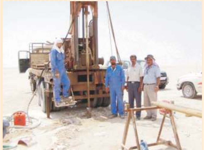
Drilling Operation in Progress in Overseas Project
