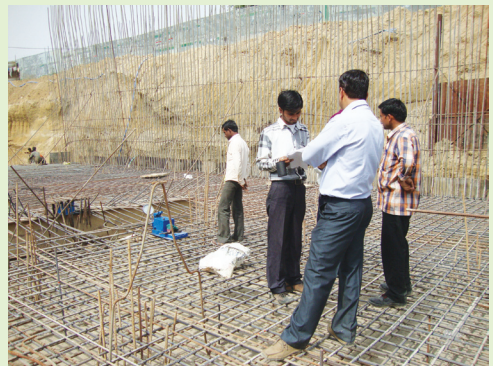
Reinforcement checking of raft being done at RUB Mundka, New Delhi
