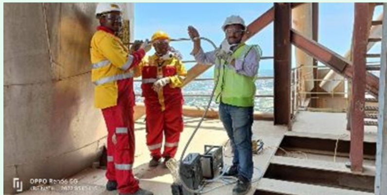
Measurement of moisture in flue gases
