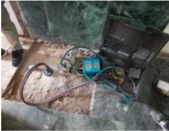
Air Permeability Test on the slab of a building structure in Delhi
