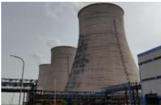
Project site of Natural Draft Cooling Towers at IGSTPP, Jharli Haryana
