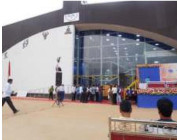
Indoor Multipurpose Hall at Vaghodia (Vadodara)
