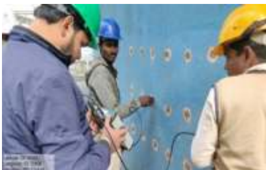
UPV testing on wall of Clariflocculator structure NTPC Singrauli
