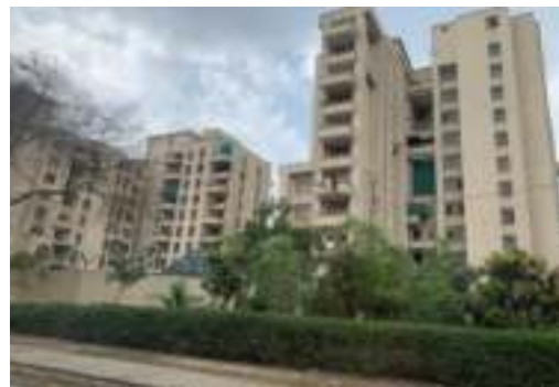
Project site of Residential Blocks at NHAJ Residential Enclave at Dwarka, New Delhi
