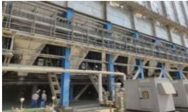
Sample Collection from ESP at one of the NTPC Plant
