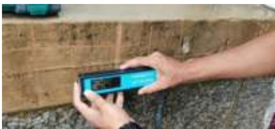
Measurement of surface electrical resistivity on an identified beam in NCB premises
