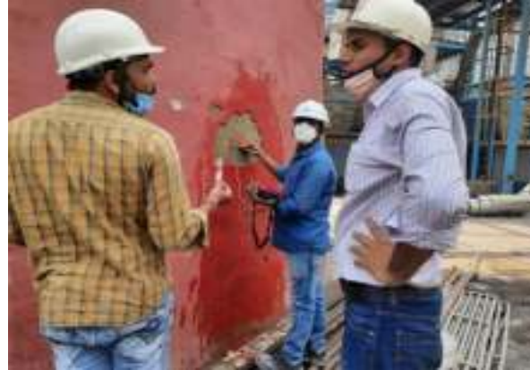
Non-Destructive Testing being carried out on RCC Chimney of NALCO, Angul, Odisha
