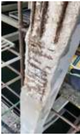
Chipping completed in a selected column at a project site
