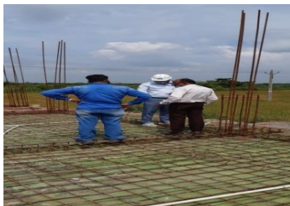
Checking of Steel Reinforcement
