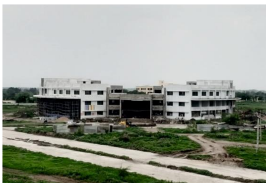
Sports Hostel at Desar
