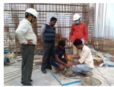
Slump test at Site
