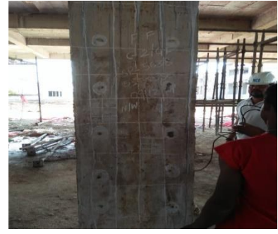
UPV Test on Concrete Column
