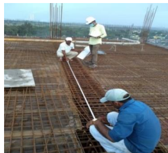
Checking of Steel Reinforcement
