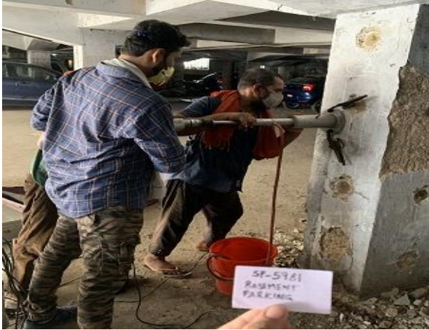
Concrete Core Extraction from Column of Parking structure
