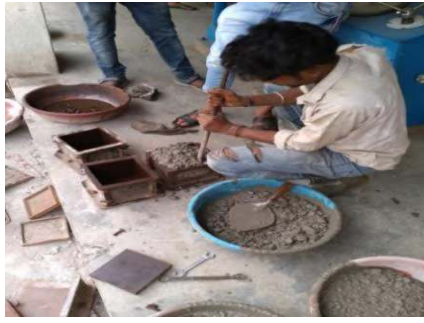
Concrete Cube filling at Site
