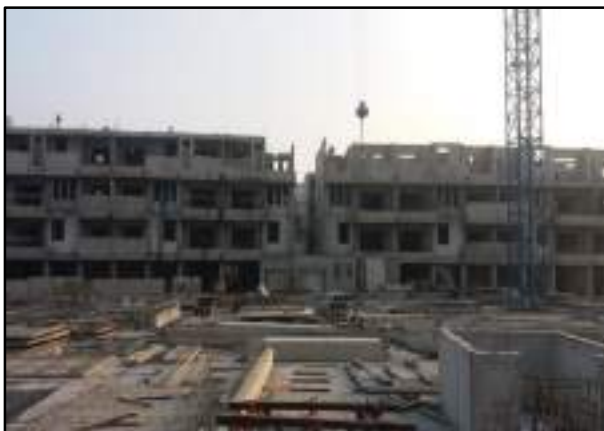
Delhi Development Authority Project, Dwarka
