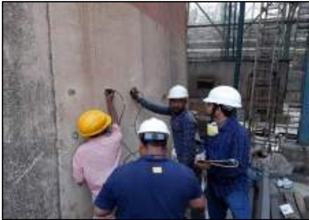
Ultrasonic Pulse Velocity test on 200m High RCC Chimney
