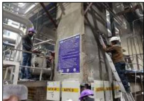
Quality assesment on TG Unit Column
