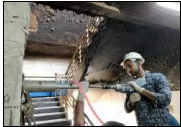
Core extraction from a Fire Damaged RCC Building
