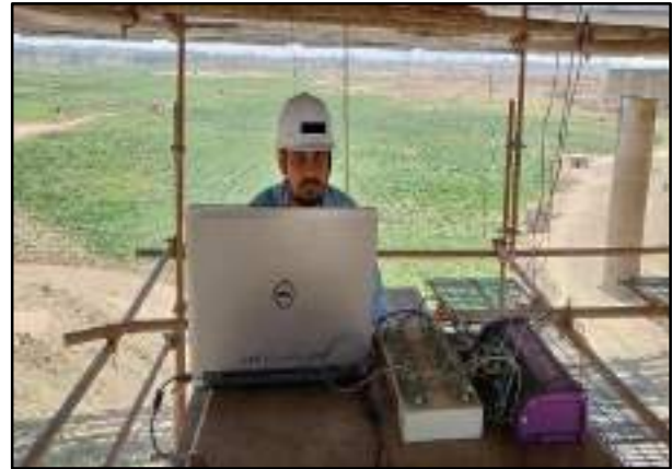
Strain measurement test on RCC girders for 400m PSC Bridge
