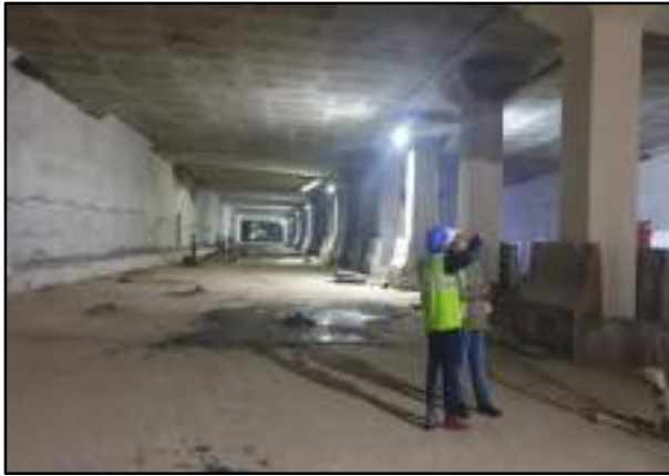
Tunnel Near Pragati Maidan (PWD/ITPO)
