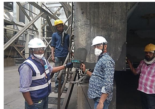
UPV testing on FD Fan foundation at NTPC Mouda
