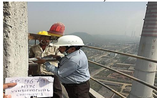
Rebound Hammer Testing on Chimney at NTPC Vindhyachal
