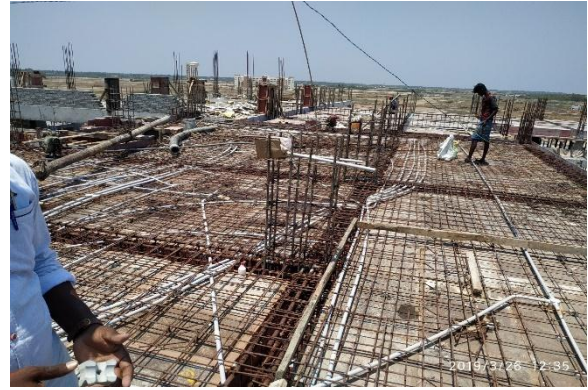
Verification of Reinforcement detailing before concreting at IISc Chellakere, Karnataka
