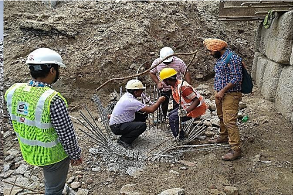
Pile Integrity test at ITPO
