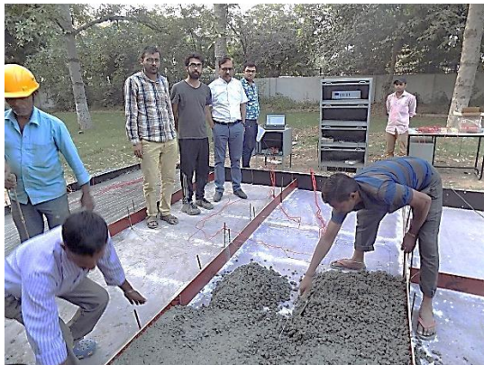
Casting of Pavement in progress
