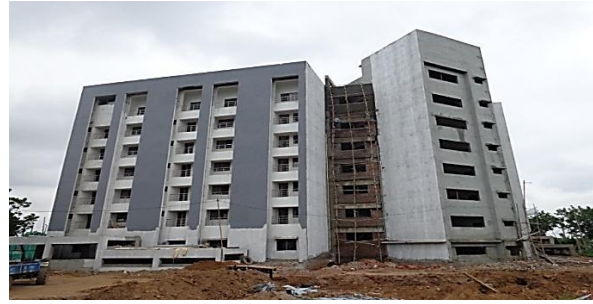
Construction of Sports Hostel at Nadiad
