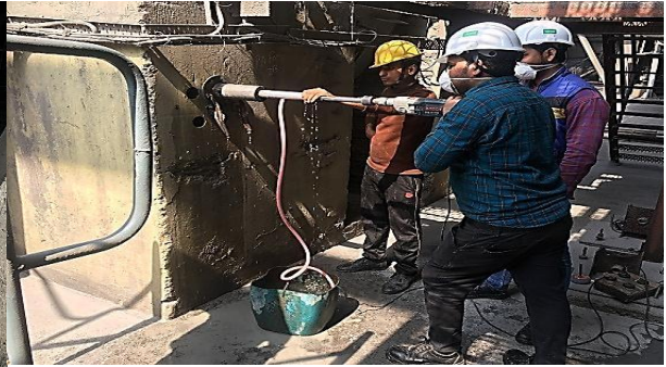
Core extraction at PA Fan Foundation at NTPC Kanti Bijlee
