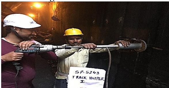
Core Extraction at Track Hopper at NTPC Dadri
