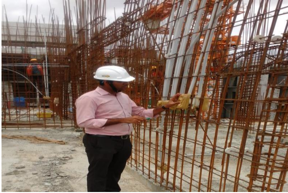
Measurement of Conduits and Switch Boards
