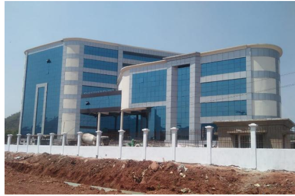
Commercial Complex at Mehisapat, Denkanal
