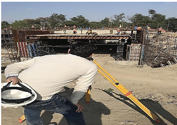
Tunnel works in Pragati Maidan
