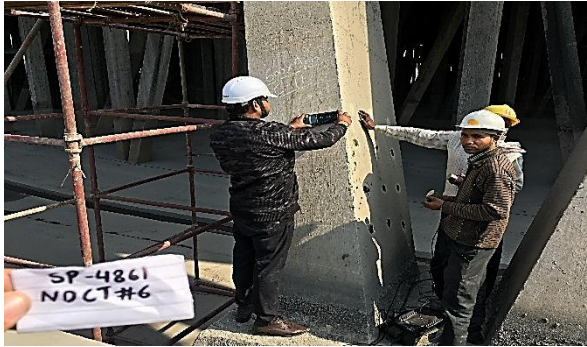
Profoscope testing at Natural Draft Cooling tower at NTPC Dadri
