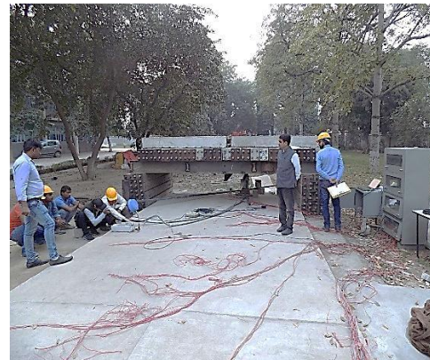
Load testing and monitoring of stresses
