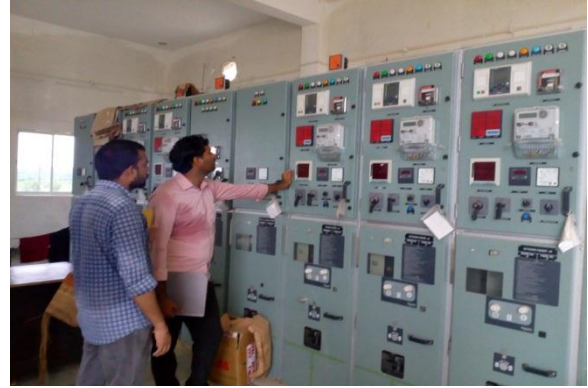
Verification of Electrical Panels
