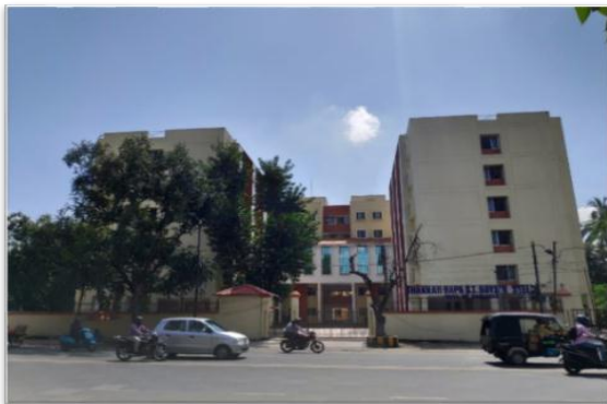
500 seated Thakarbapa Hostel Building, Bhubaneswar
