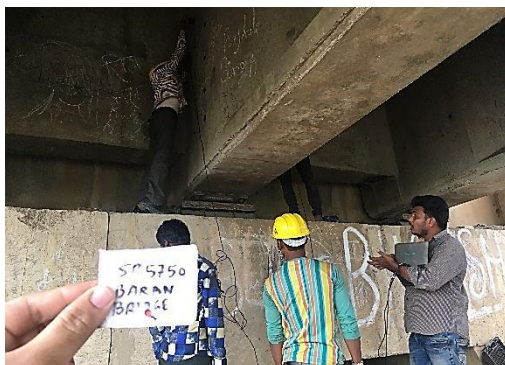
UPV testing on MGR Bridges at NTPC Rihand
