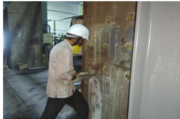
Rebound Hammer Testing being done on RCC Column of TG Unit#1 of NTPC Unchahar
