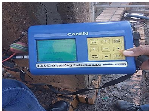
Half-cell Measurement test on Bulk Storage Tank at NTPC Jhanor
