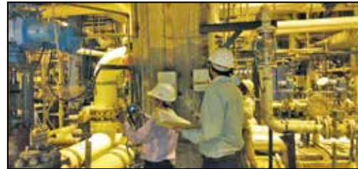
UPV testing on RCC Column of TG Unit Capacity 500MW at NTPC
