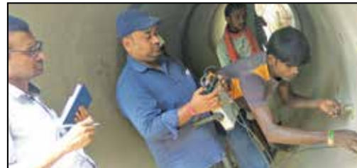
UPV Testing for 2200mm Diameter RCC Pipe Line at Varanasi
