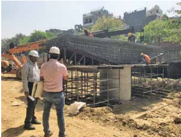
Inspection of Flyover project at Barapulla
