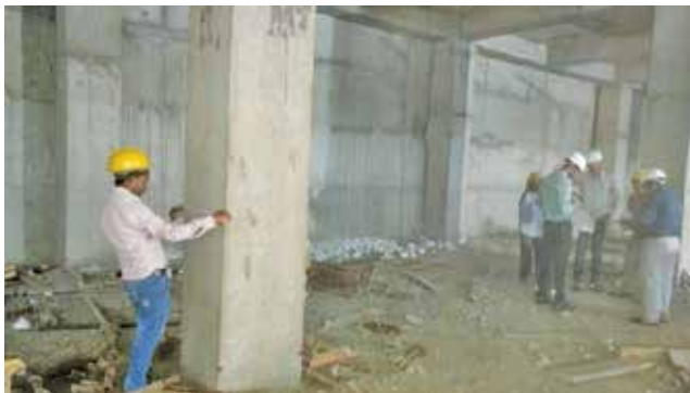
NDT at Western Court Annex MP Hostel, Janpath
