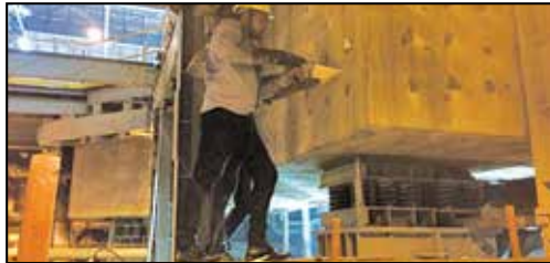
Extraction of Concrete Powder sample from TG Deck Slab
