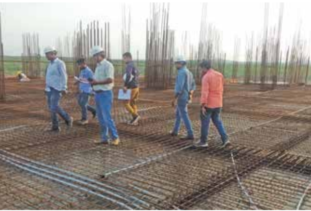
Checking Reinforcement at Incubation Centre, IDCO
