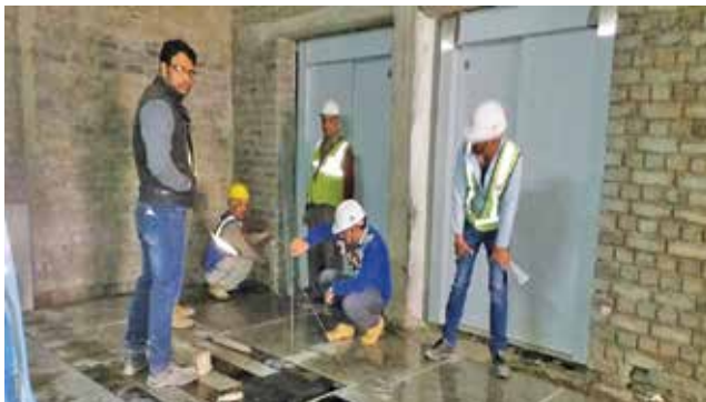
Floor Level checking at AIIMS
