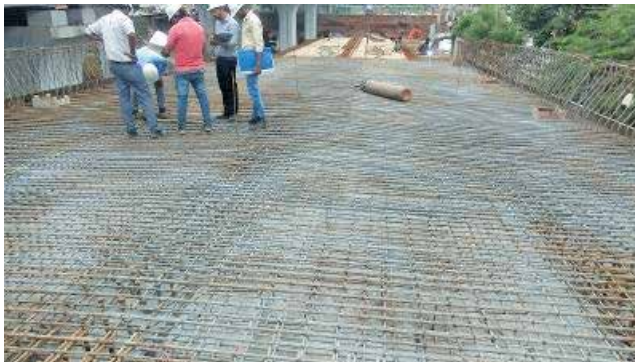
Checking Reinforcement at Flyover, Barapulla
