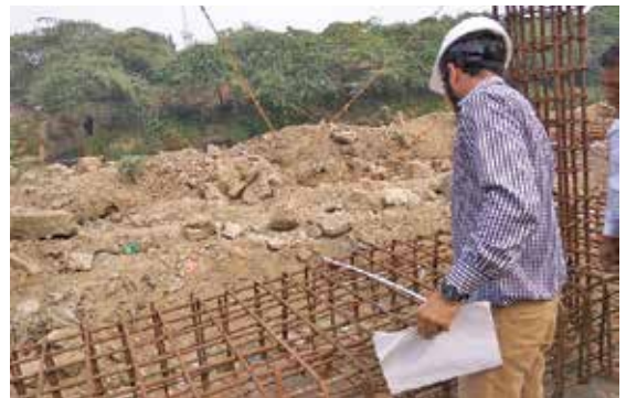
Checking Reinforcement at Strip Footing of Recreation Centre
