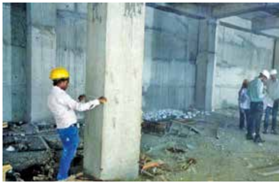
Non-destructive Testing at Western Court Annexee MP Hostel, Janpath
