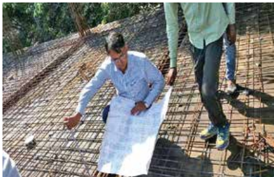
Checking of Reinforcement of Slab at School site
