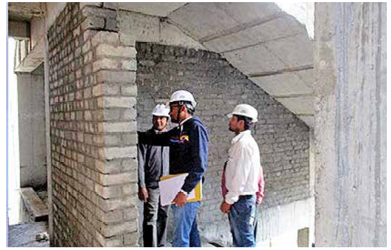
Inspection of Brick Work at President's Estate Project
