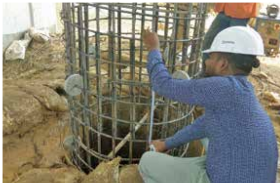
Checking Reinforcement of Pile at Flyover Project at Barapulla
