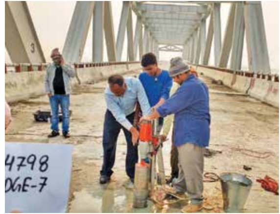
Extraction of Core from Bridge Deck Slab at EC Railway, Patna
