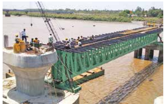
Inspection of Pier at Pedestrian Bridge Project
