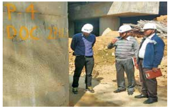
Inspection of Pier at Flyover Project at Barapulla
