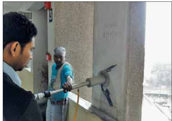
Extraction of Concrete Core from RCC Column of OFOCGHS, Dwarka, Delhi
