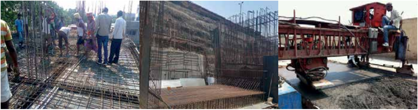
Slab Casting of SDMC Underpass at Bijwasan, Delhi
