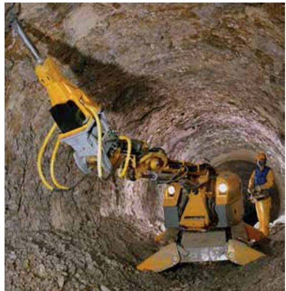
Demolition of Old Lining using De-bricking Machine
