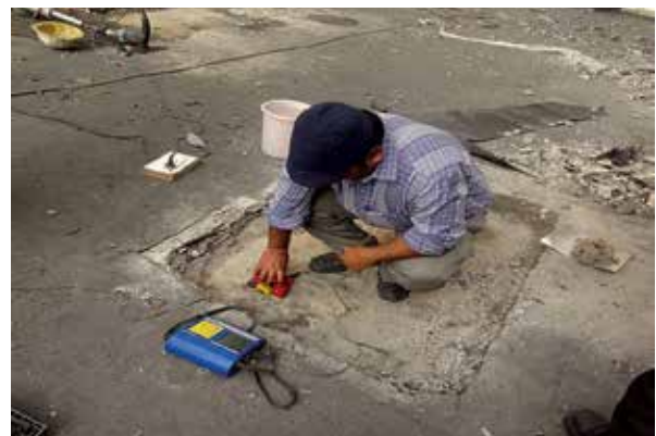
View of Ferro Scanning Examination at NTPC, Vindhyachal
