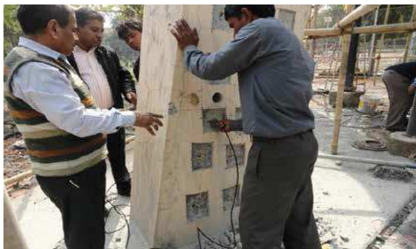
UPV testing of column of water tank at RBI Bhopal
