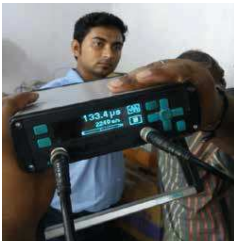
View of ultra sonic pulse velocity test on column of community centre building at Faridabad
