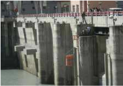
View of up-stream side of the Nathpa Dam
