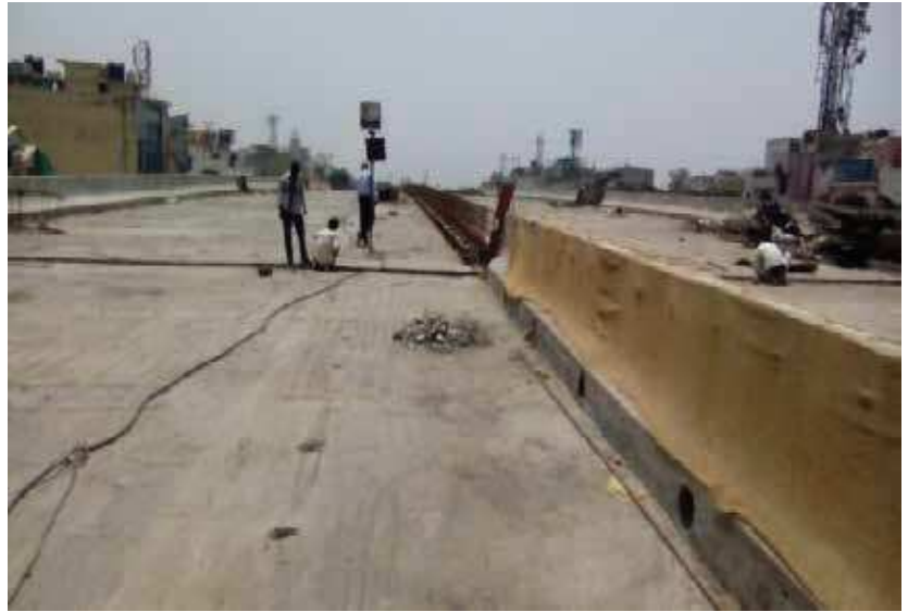
NCB engineers at TPQA project site of PWD, Vikaspuri flyover, Delhi
