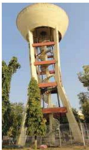
View of overhead tank at RBI Bhopal
