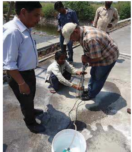
Extraction of Concrete core Samples from Bridge Deck
