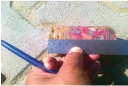
Carbonation depth being measured on extracted concrete core sample
