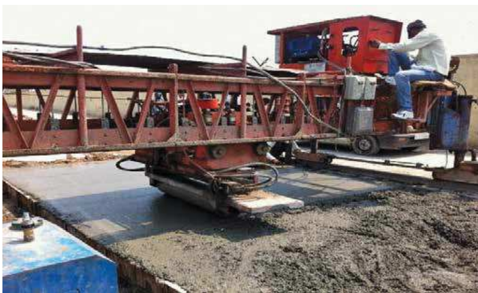
MCD Road Work at Okhla, Delhi
