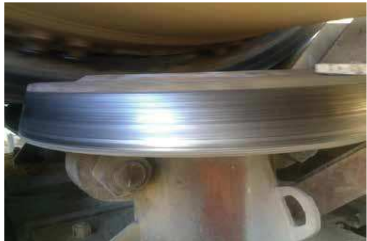
View of Aggressive Scoring Developed on the down hill side of the Thrust Roller of Kiln - 1
