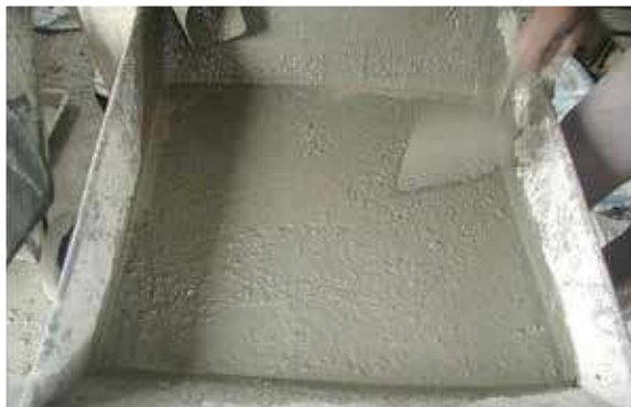
Self Compacting Concrete
