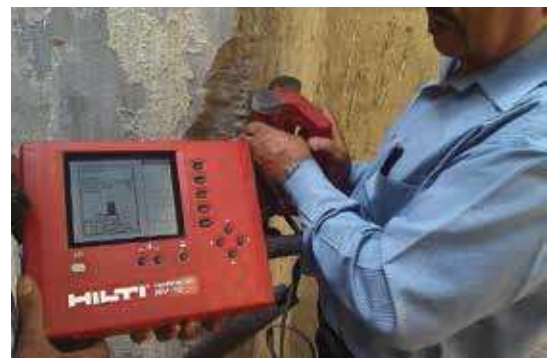
Reinforcement location and cover thickness being assessed by Ferro Scanning Technique
