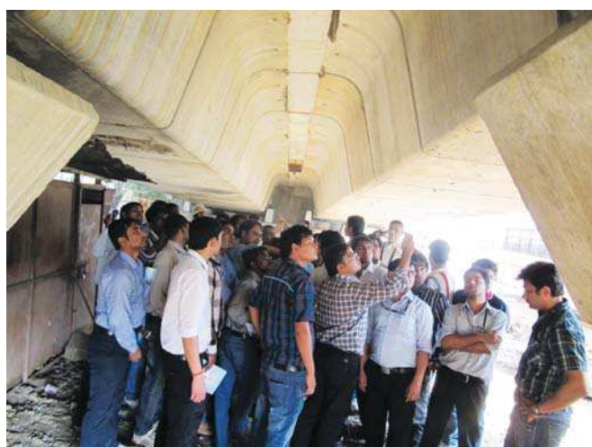
Trainees is being given demonstration on a construction site
