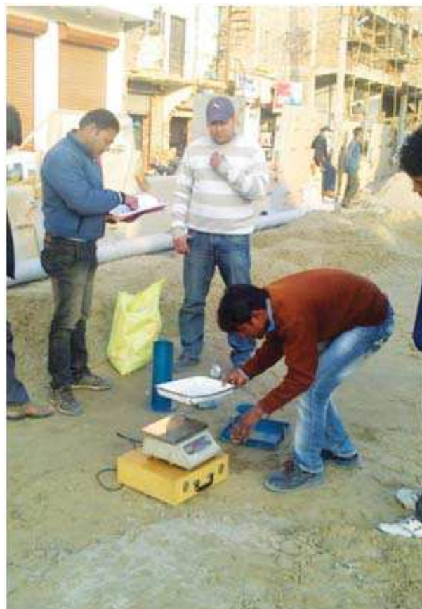
Compaction Test by Sand Replacement Method at a ROB in Delhi
