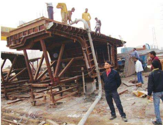
Segment Casting being Supervised at a Casting Yard
