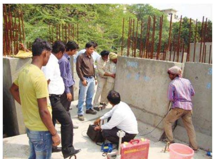
UPV test on a Pre-cast segment of a drain
