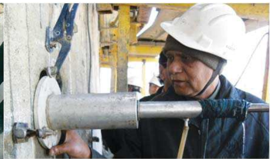
Core extraction from a RCC Chimney
