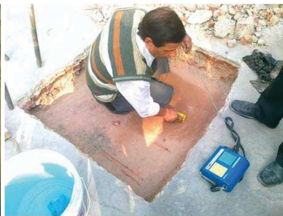
Scanning of reinforcement before extraction of core sample
